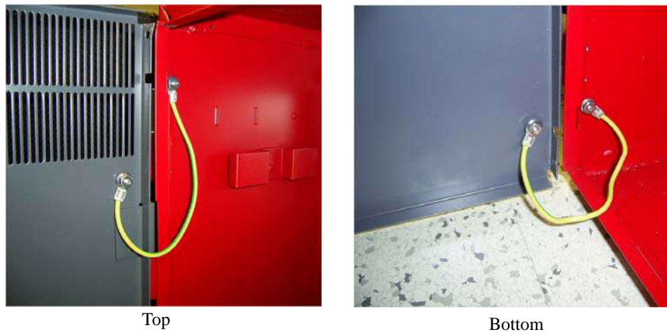
Figure 5-3. Dead front grounding straps
